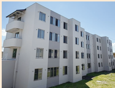
寮棟(1棟)外観 Exterior of Dormitory
